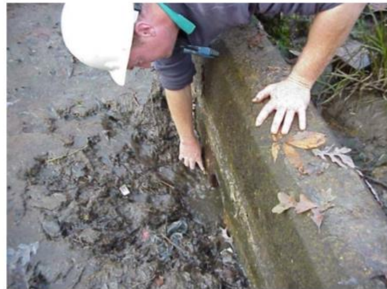
Figure M2.3: After clog is removed.
