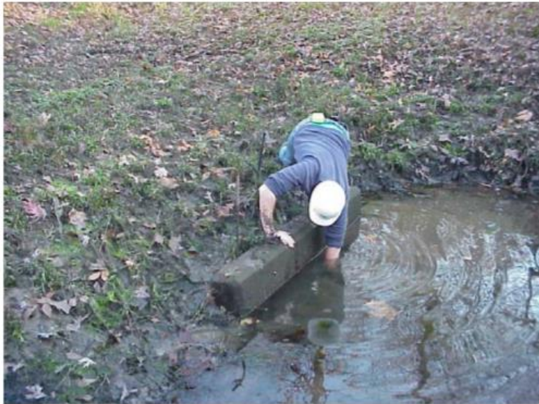
Figure M2.2: Clogged low flow orifice (before maintenance).
